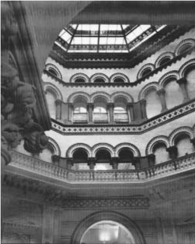
Fig. 3. Restored rotunda. The key to the fire-management plan was the restoration of the rotunda for use as a smoke reservoir. In the event of fire, smoke and combustion gases are collected in the upper section of the rotunda, above and below the stained-glass laylight. The arched openings at the upper level were filled in with heat-resistant glass panels. Fans at the attic level extract smoke directly to the exterior, making the connecting corridors and staircases safe egress routes. Photograph by Michael Rogol.
