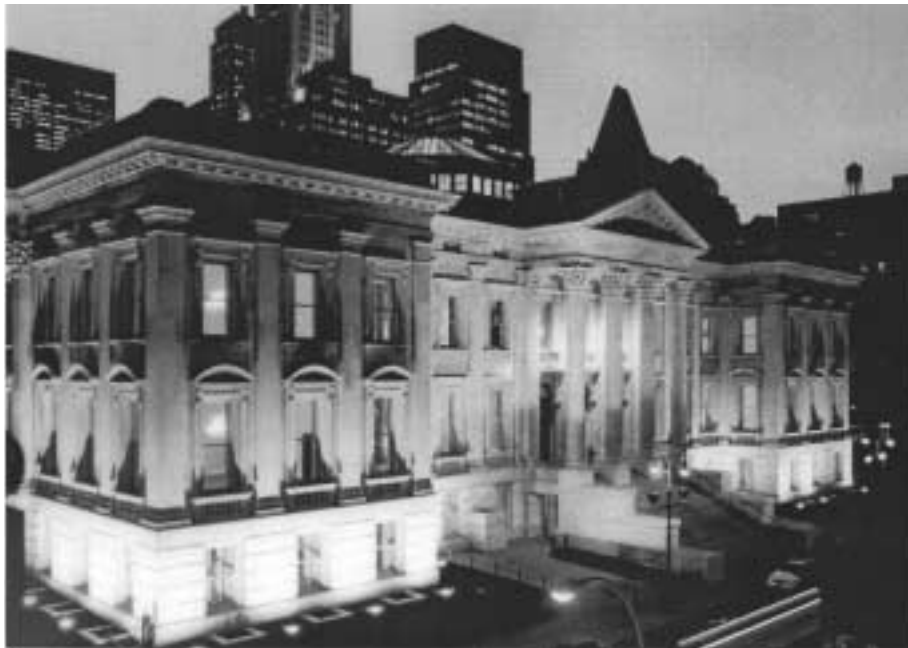
Fig. 1. Tweed Courthouse, 52 Chambers Street, New York City, restored exterior. The exterior of the courthouse, constructed of Tuckahoe and Sheffield marbles, was completely restored. More than 1,500 pieces of stone were repaired across the entire building facade. The entire 1,220-foot-long cornice, including 335 modillions, was replaced. The monumental Chambers Street stairway, which was removed in the 1940s for street widening, was rebuilt as the main entrance to the building. Along with the re-establishment of the three double-doorway entrances on the main floor, the restored stairway provides code-complying egress for the new uses of the building. Previously, the building did not have adequate egress and exiting. Photograph by Michael Rogol.
