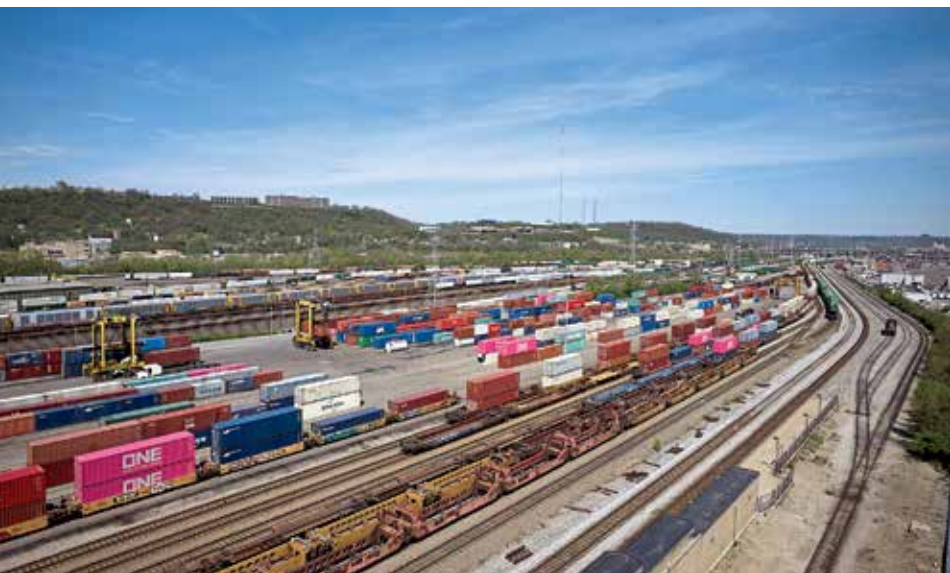
The railyard behind Union Terminal is now owned and operated by CSX Transportation.
